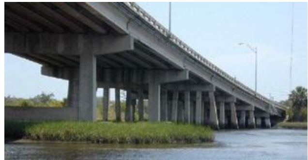
San Pablo River bridge Jacksonville Fl. – steel hardware
